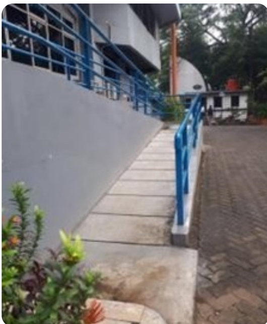
Ramp di setiap gedung Ramp in every building
